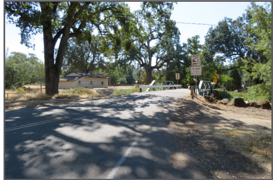
Figure 4.17: Narrow bridge with no space for walking in Paynes Creek.
