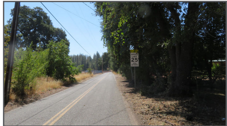
Figure 4.18: Lack of shoulders for students to walk or bike, and overgrown school zone sign.
