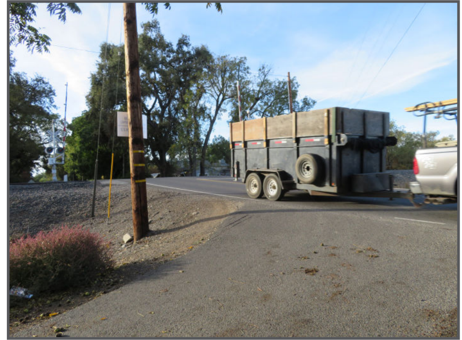
Figure 4.20: Unsafe conditions at an intersection in the City of Tehama due to proximity of RR tracks, lack of shoulders, ditches at sides of roadways.
